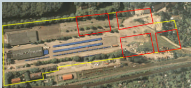
Bird's eye view of the Alte Wöhr construction site
