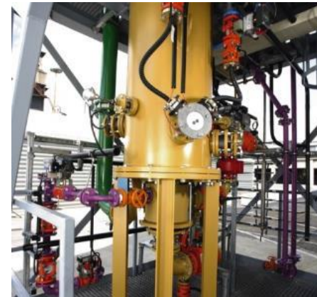
Bottom burner section of HCl synthesis unit
