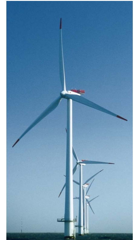
Offshore wind farm
