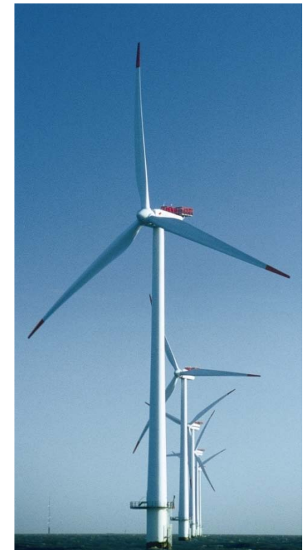
Offshore wind farm
