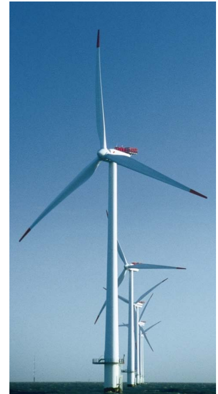
Offshore wind farm
