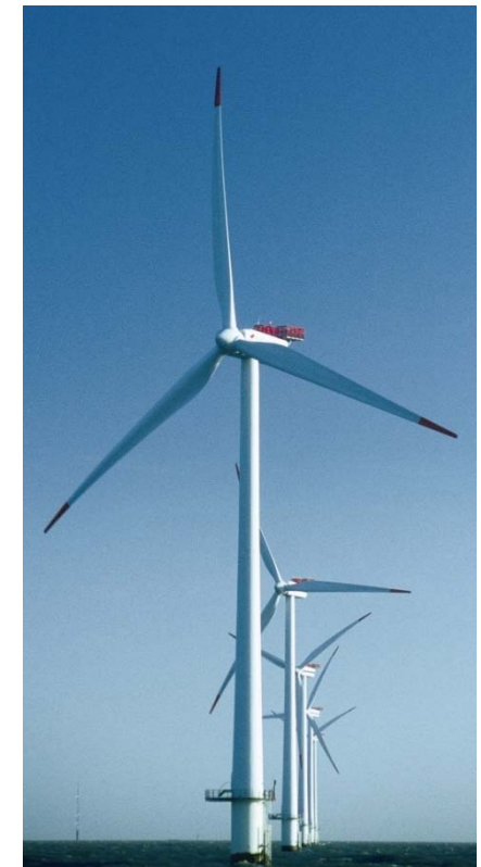
Offshore wind farm
