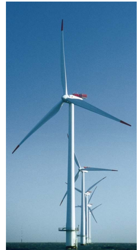
Offshore wind farm
