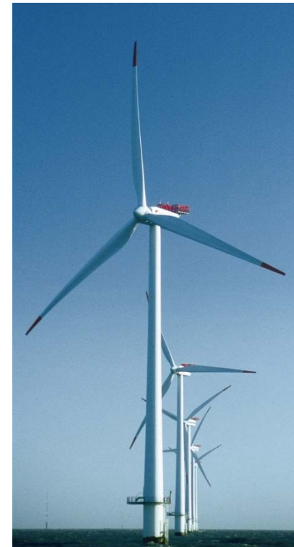
Offshore wind farm
