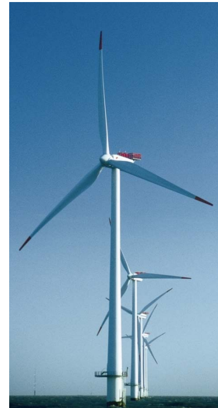
Offshore wind farm
