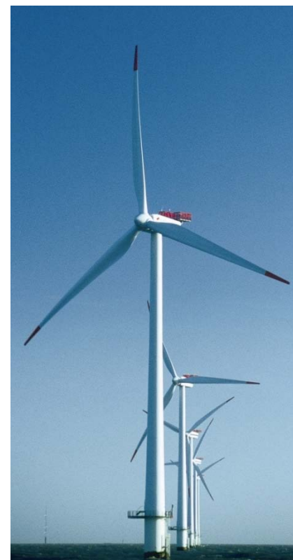
Offshore wind farm
