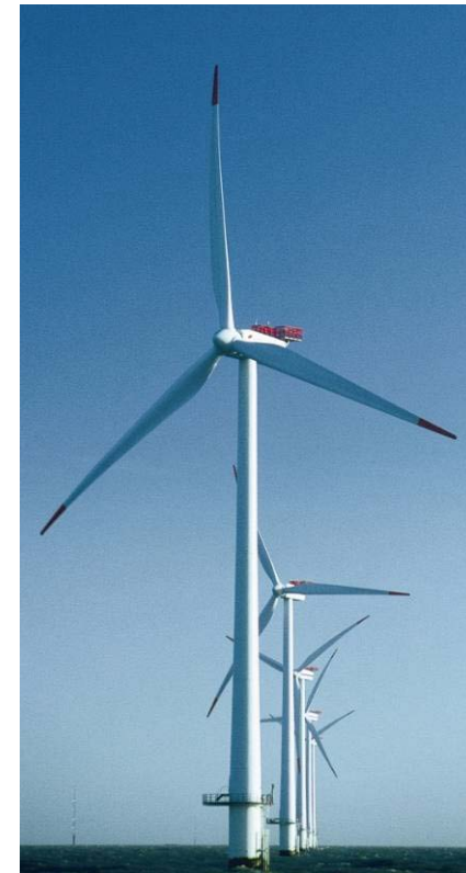
Offshore wind farm
