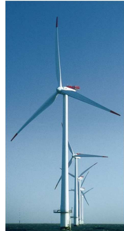
Offshore wind farm
