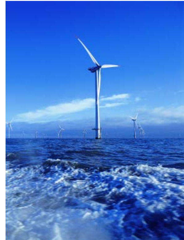
Offshore wind farm
