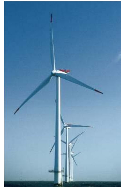
Offshore wind farm
