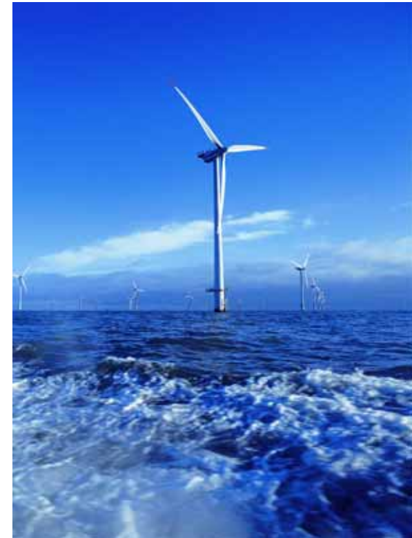
Offshore wind farm
