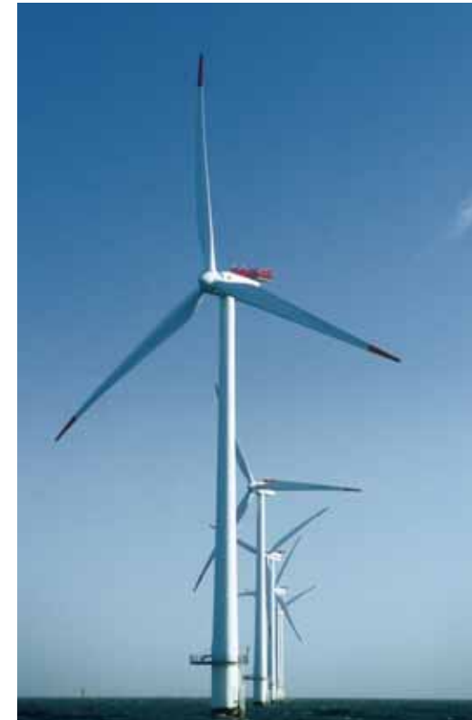
Offshore wind farm
