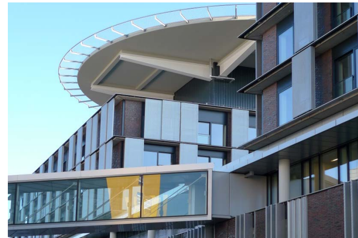
Technical Service Contract – University Medical Center Hamburg-Eppendorf
