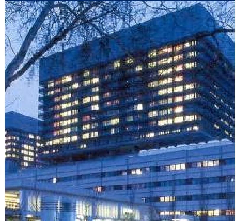
Largest service business contract – University Hospital AKH Vienna
