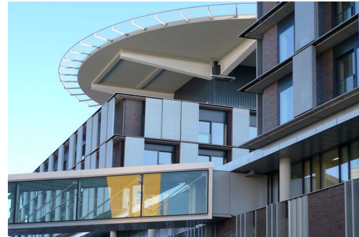
Technical Service Contract – University Medical Center Hamburg-Eppendorf
