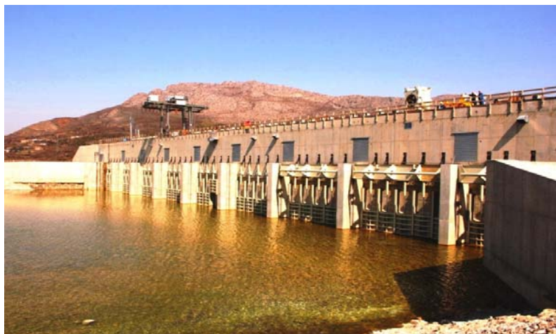
Project Ashta on the Drin River
