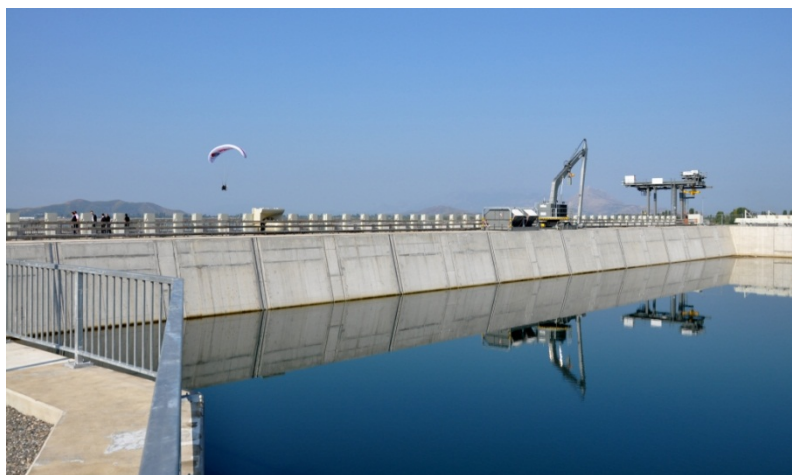
Project Ashta on the Drin River
