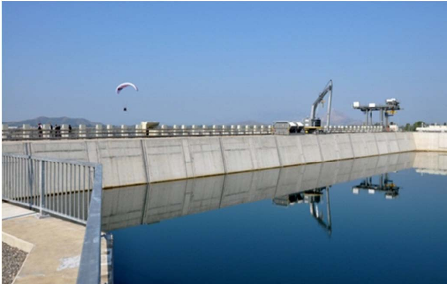
Project Ashta on the Drin River
