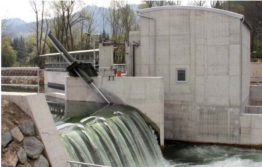
Small-scale hydropower plant Schaldorf
