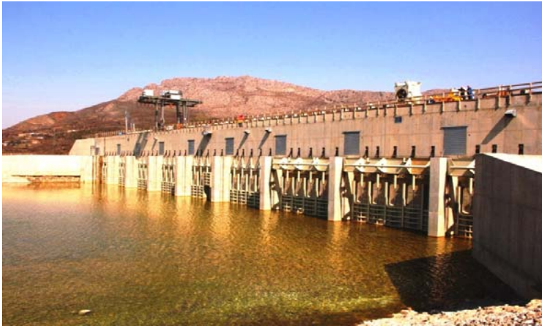
Project Ashta on the Drin River
