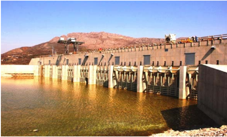
Project Ashta on the Drin River
