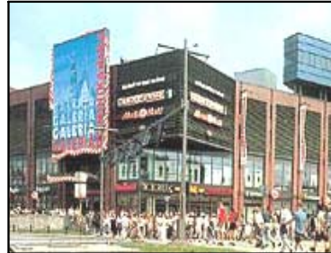
Galeria Dominikanska Wrocław, Poland
