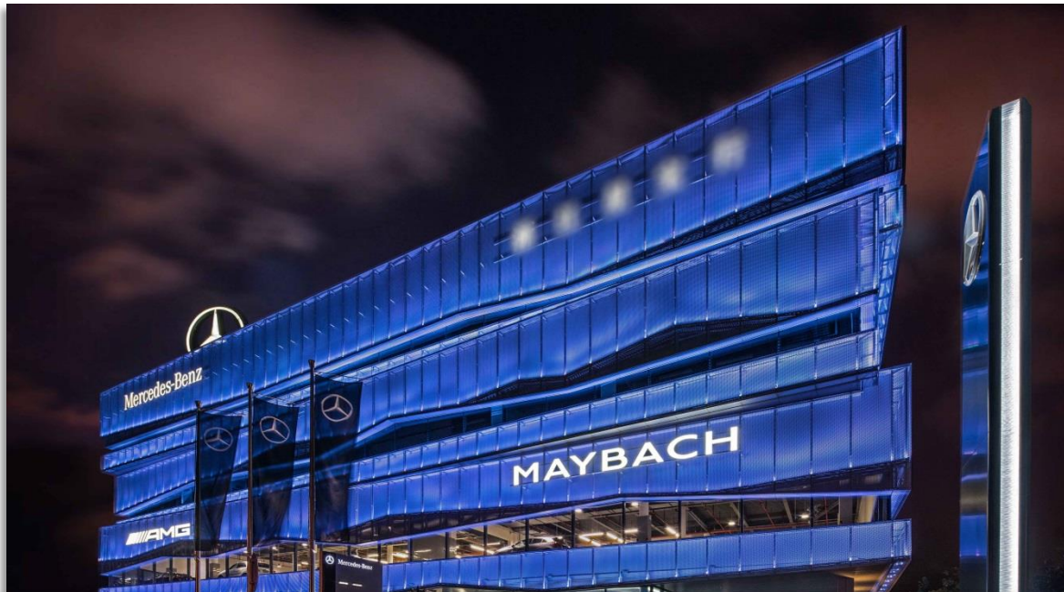
Upgrading and relocations to enhance capacities
