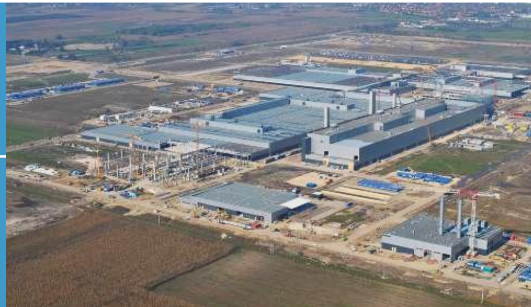
New plant in Kecskemét, Hungary
