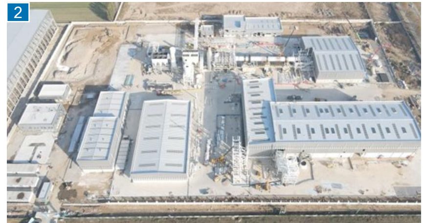
↑ Xuchang construction site, mid-November 2021
