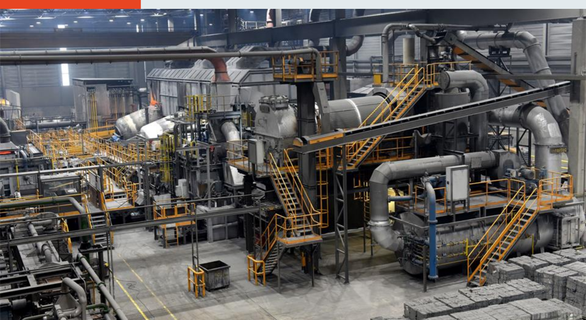
Secondary aluminium production plant at Bernburg, Germany
