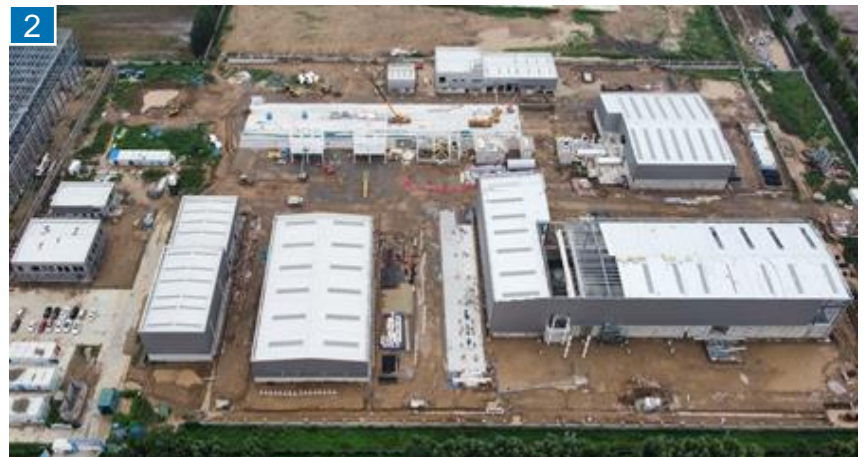
↑ Xuchang construction site, mid-August 2021
