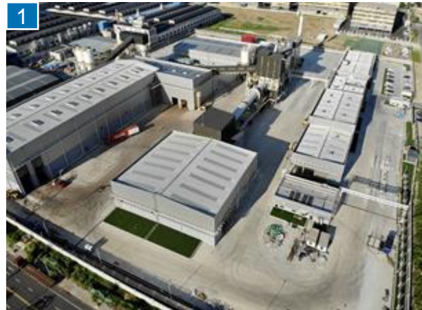
↑ Changzhou plant, completed
