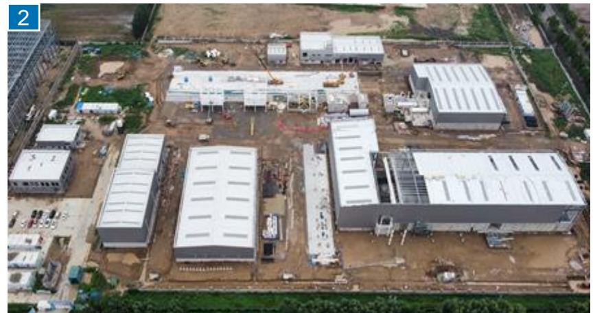
↑ Xuchang construction site, mid-August 2021
