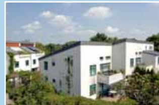
Kieselbronner Weg 52 residential units 1990s
