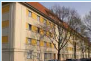
Togostraße 370 residential units 1920s to 1940s
