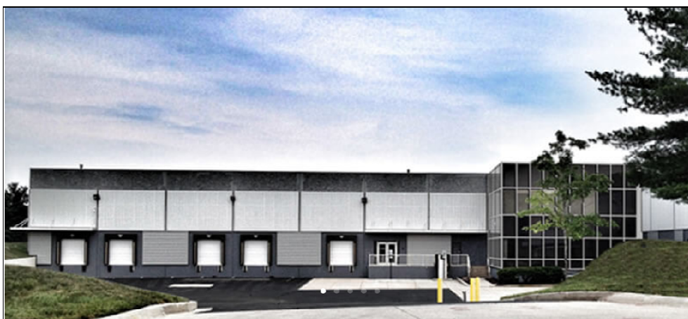
Figure 1: State of the art production facility in Baltimore, Maryland, USA
