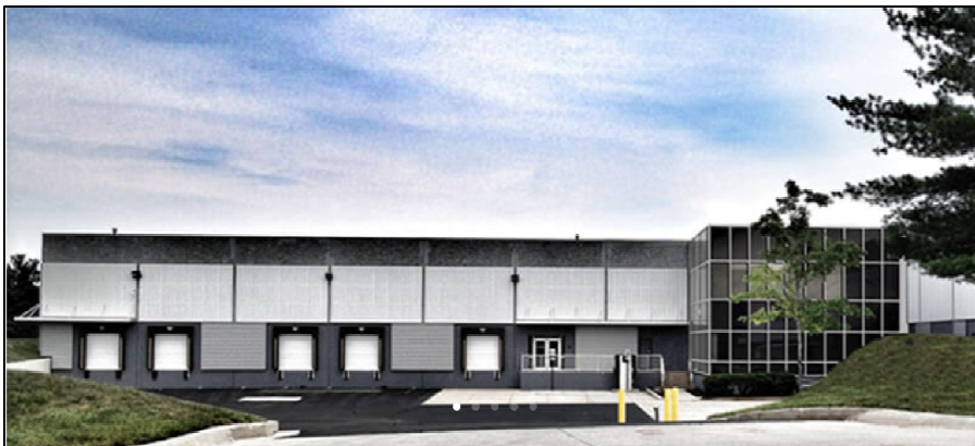
Figure 3: State of the art production facility in Baltimore, Maryland, USA
