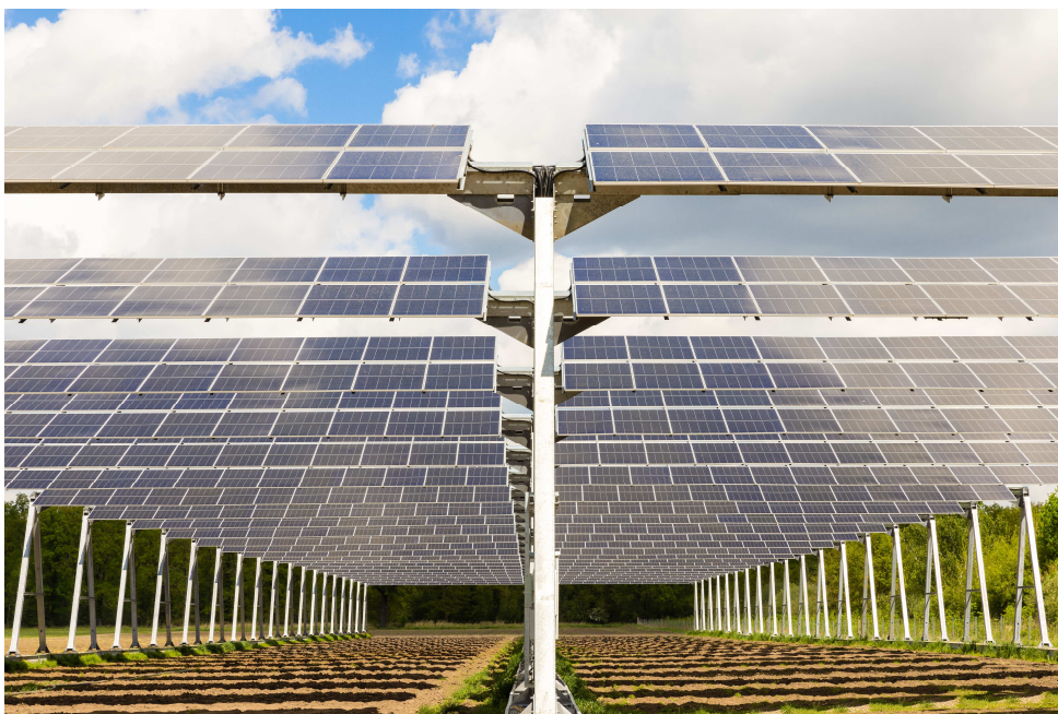
Figure 3: Solving scarcity of farmable dirt with agrophotovoltaics
