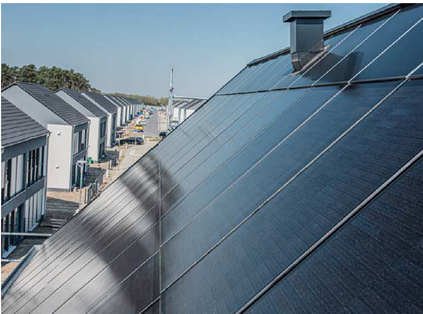
Figure 8: Ludwigsfelde building project
