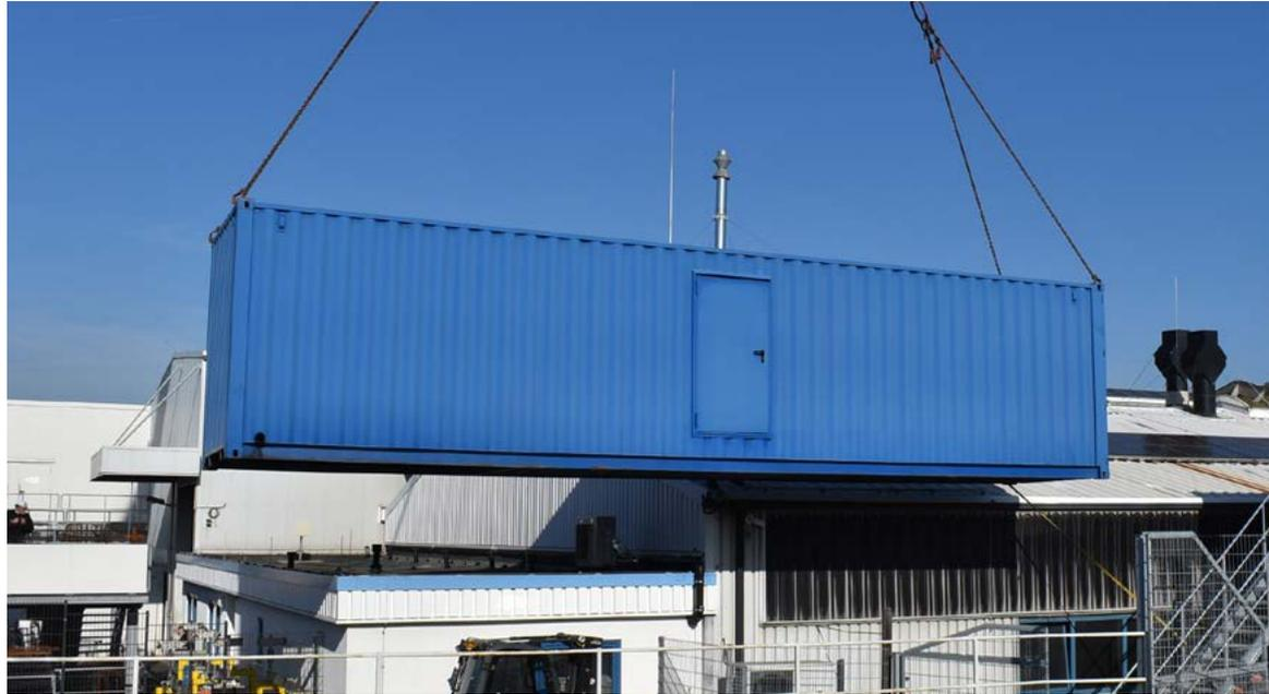
Installation of the biofilter in container form.
