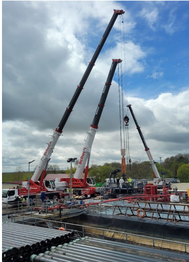
Figure 1: Natürlich Insheim - Pump replacement works.
